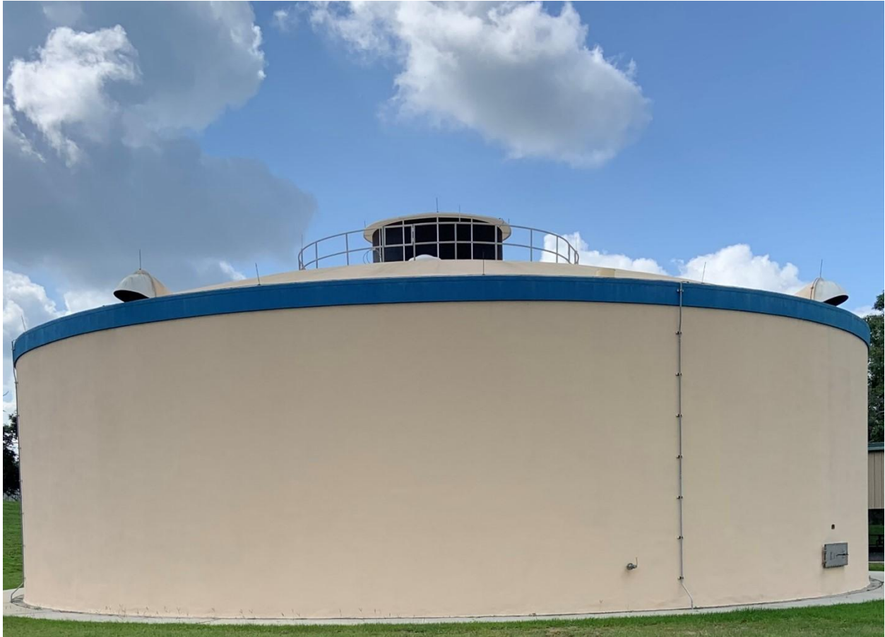
Figure 1 Cherry Hill Water Treatment Facility.
