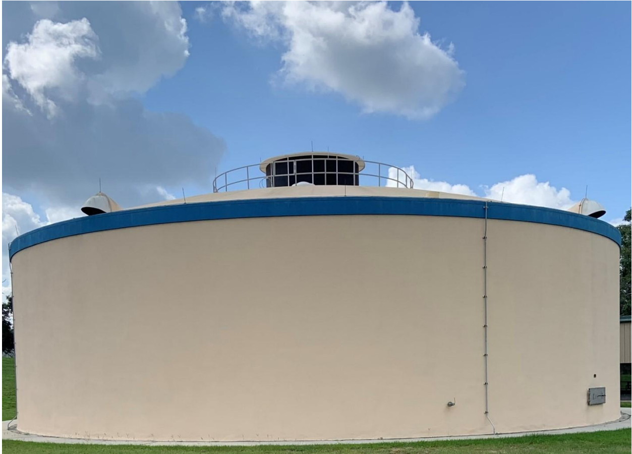
Figure 1 Cherry Hill Water Treatment Facility.
