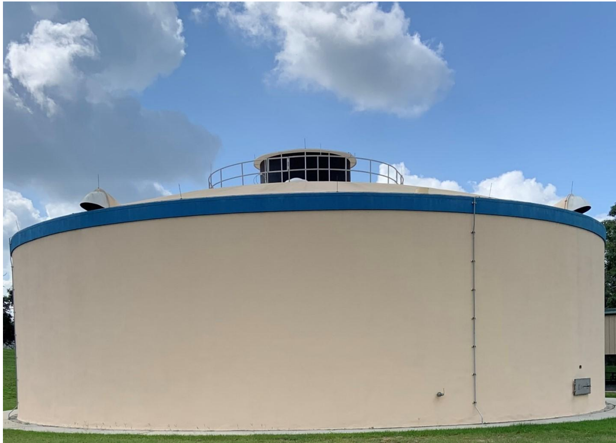
Figure 1 Cherry Hill Water Treatment Facility.
