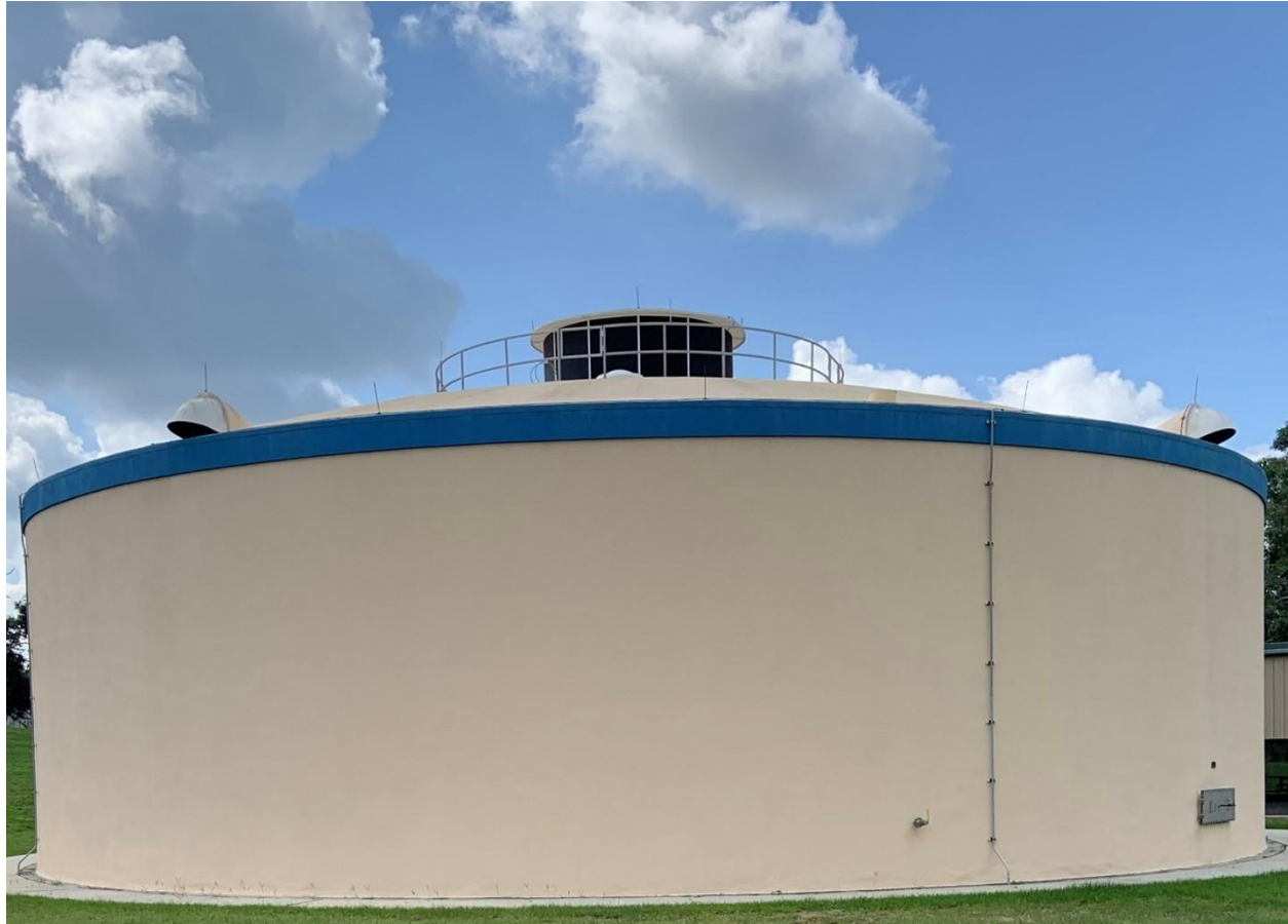
Figure 1 Cherry Hill Water Treatment Facility.
