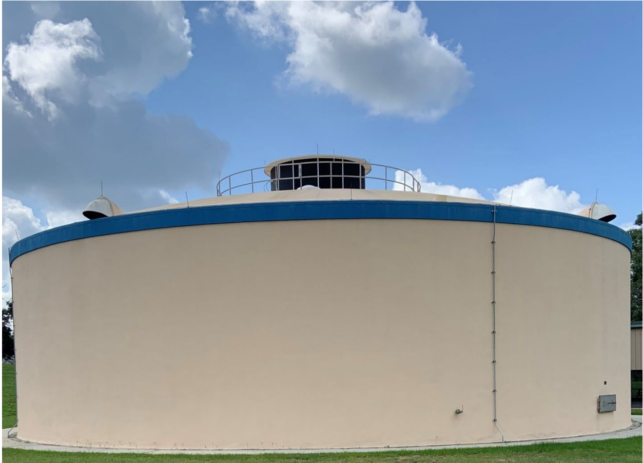
Figure 1 Cherry Hill Water Treatment Facility.
