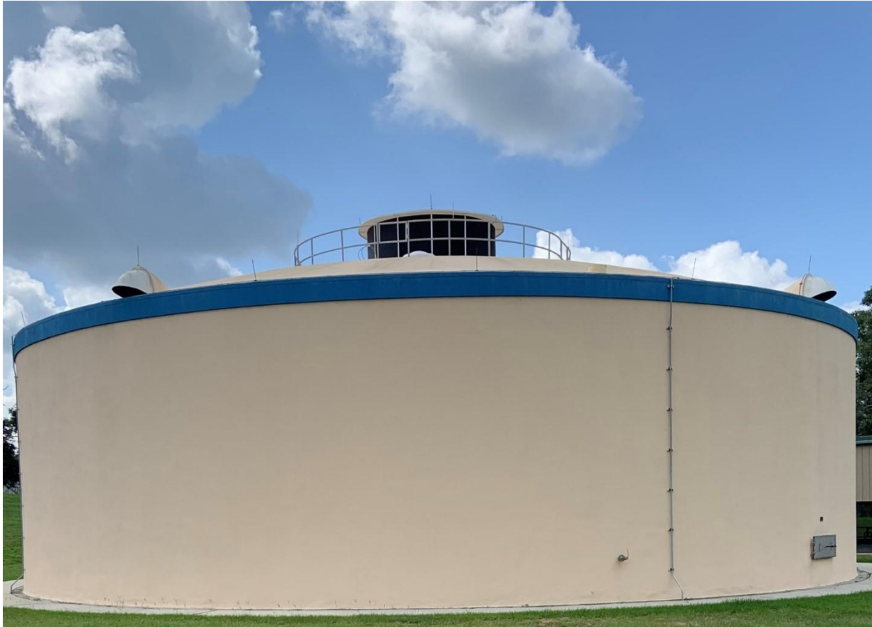
Figure 1 Cherry Hill Water Treatment Facility.
