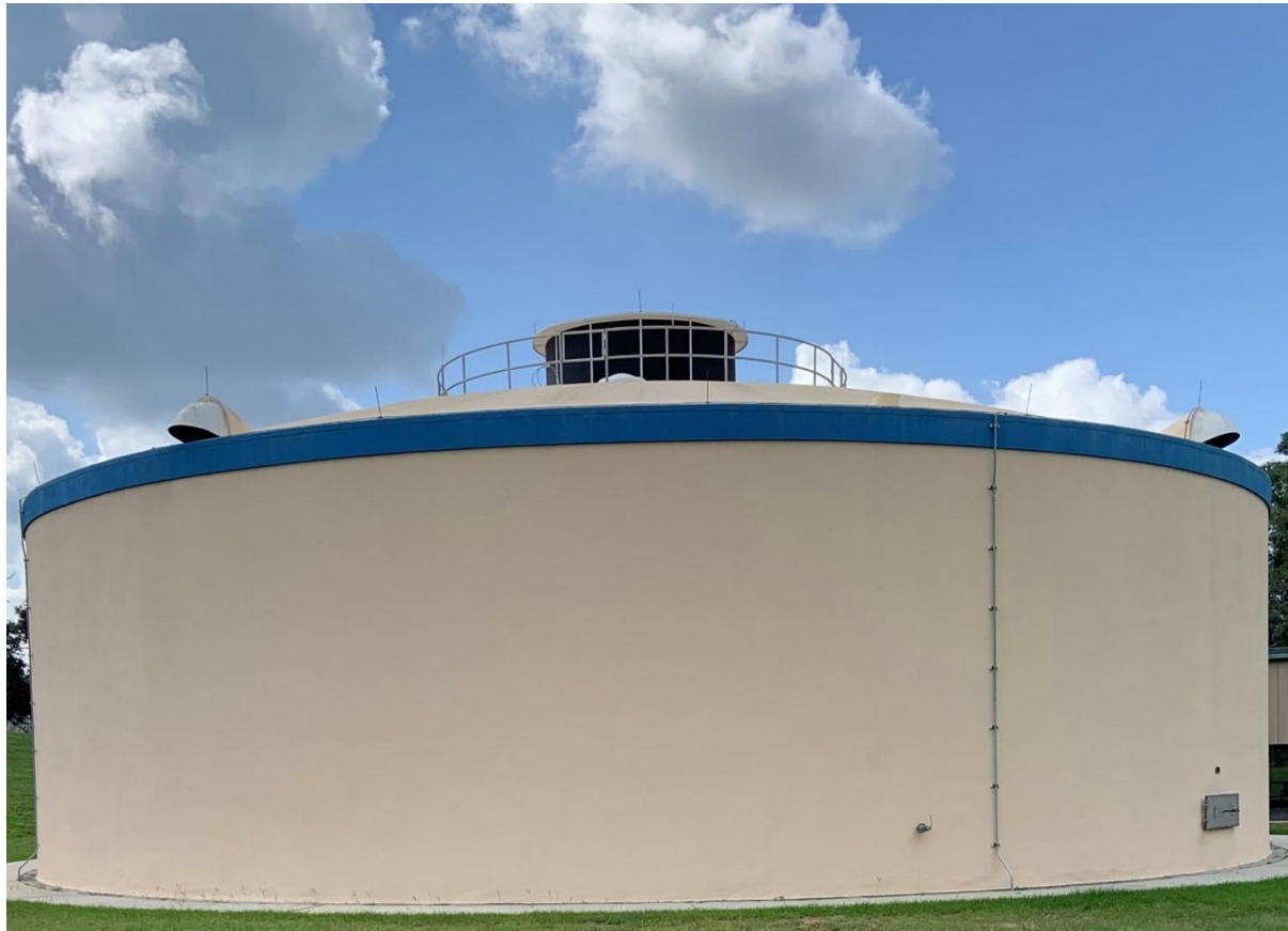
Figure 1 Cherry Hill Water Treatment Facility.
