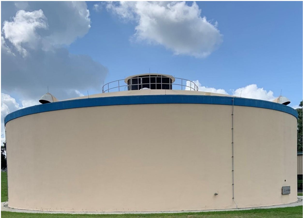
Figure 1 Cherry Hill Water Treatment Facility.
