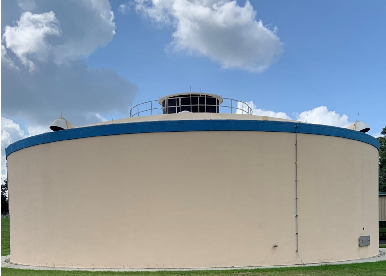
Figure 1 Cherry Hill Water Treatment Facility.
