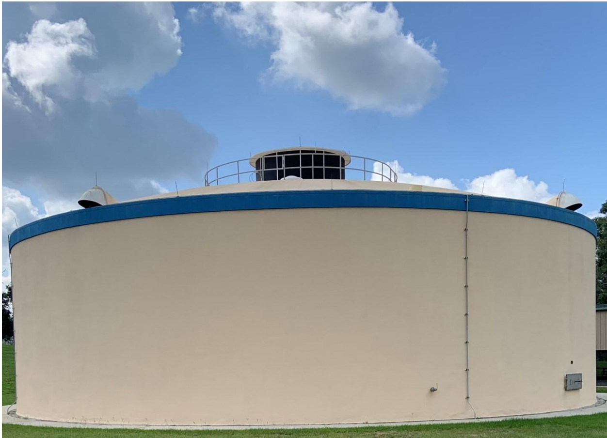
Figure 1 Cherry Hill Water Treatment Facility.
