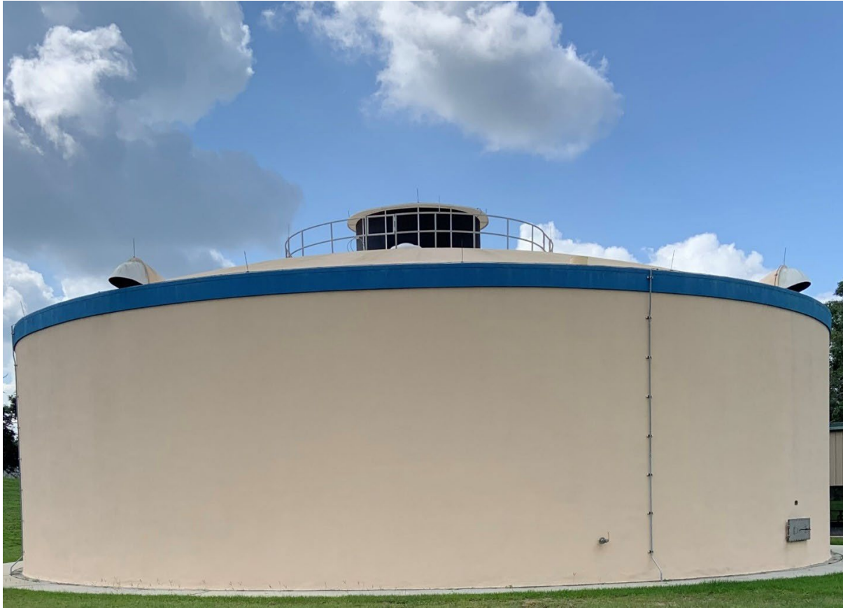
Figure 1 Cherry Hill Water Treatment Facility.
