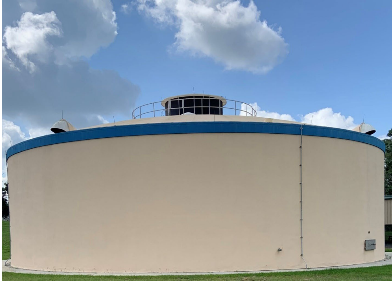
Figure 1 Cherry Hill Water Treatment Facility.
